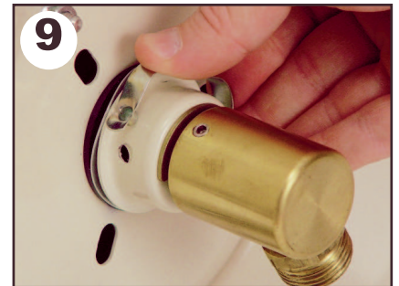
9 Push snap button onto bell cap.
